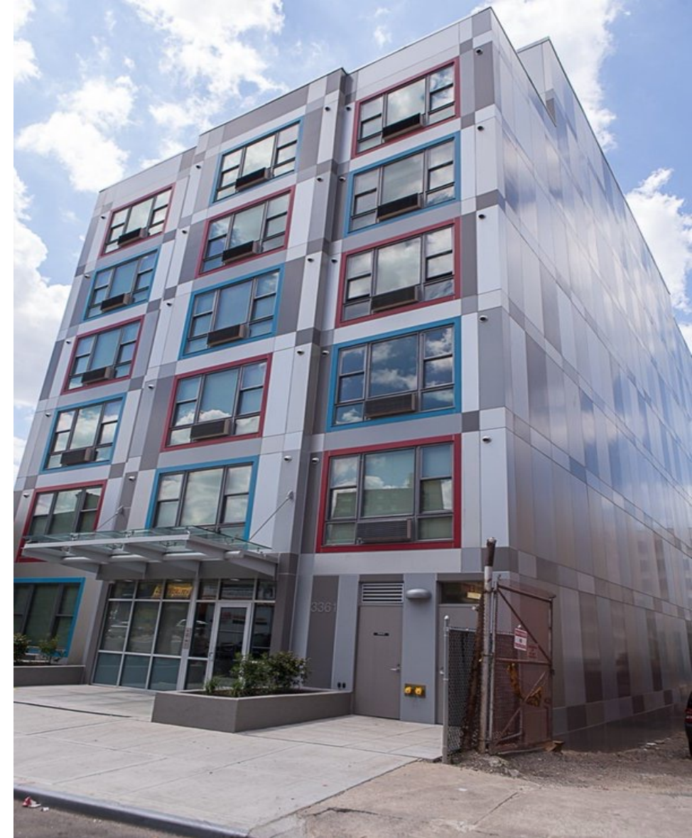
3361 Third Avenue in the Morrisania neighborhood of the South Bronx.
